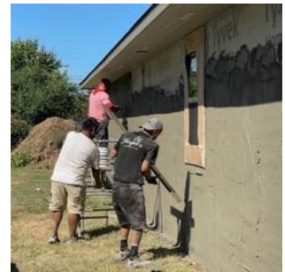
Stucco being applied to our accessory building
