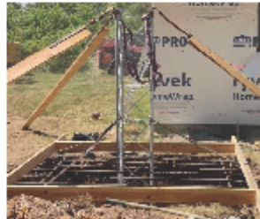
Tower base sitting in a 4 ½ foot pit with rebar waiting for concrete
