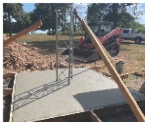
Concrete pad immediately after being smoothed and finished
